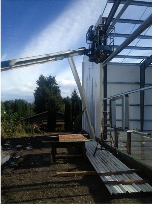
the last panel by holding the panel at a slight angle so the bottom is locking in first and the top of the panel is 6"-12" away from the eave strut at the top of the wall (this prevents it from sticking to the tape before it is locked properly).
