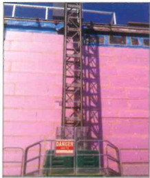
Exterior walls - Insulation to concrete
