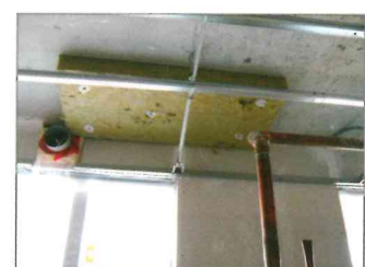
Ceiling acoustical insulation
