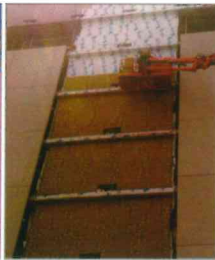
Exterior walls - Insulation to concrete
